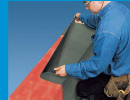
4 Install the peel and stick base flashing membrane over primed substrate.
