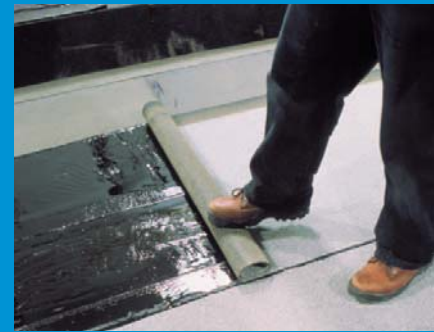
5 Apply the cap sheet in a full bed of adhesive.
