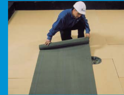
1 Unroll each roll dry for proper alignment, prior to installation.
