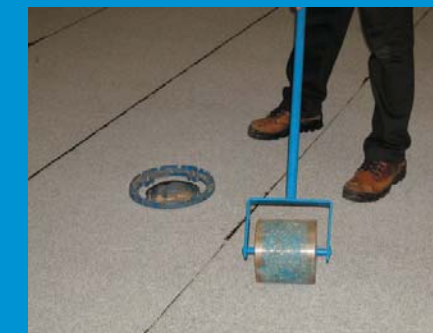
6 Roll the cap sheet to maximize adherence and eliminate voids.
