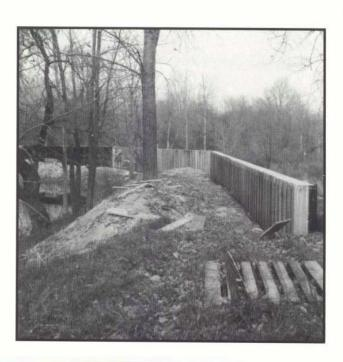
The ABILITY FORM/ELASTIZELL EF Wall is anchored with reinforcing steel to the Class VI ELASTIZELL EF footing. This reduces the uplift potential as well as lessens future settlements over the poor subsoils at this site.
