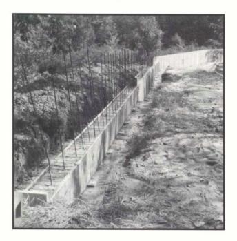
The ABILITY FORM WALL is erected quickly and filled with Class IV **ELASTIZELL EF**.
