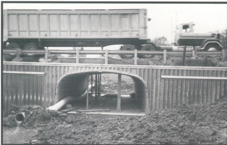
Traffic maintained, by-pass not required
