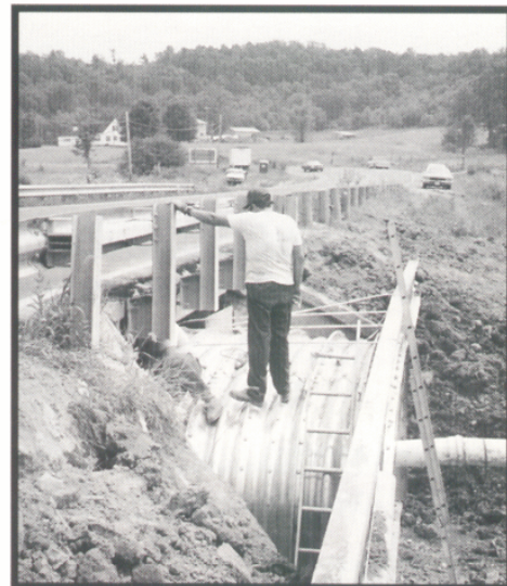
Extending width of bridge
